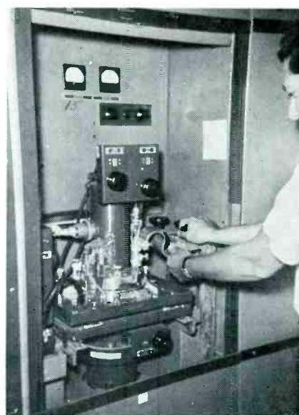
A regular program of tightening high current and RF connectors is wise.
