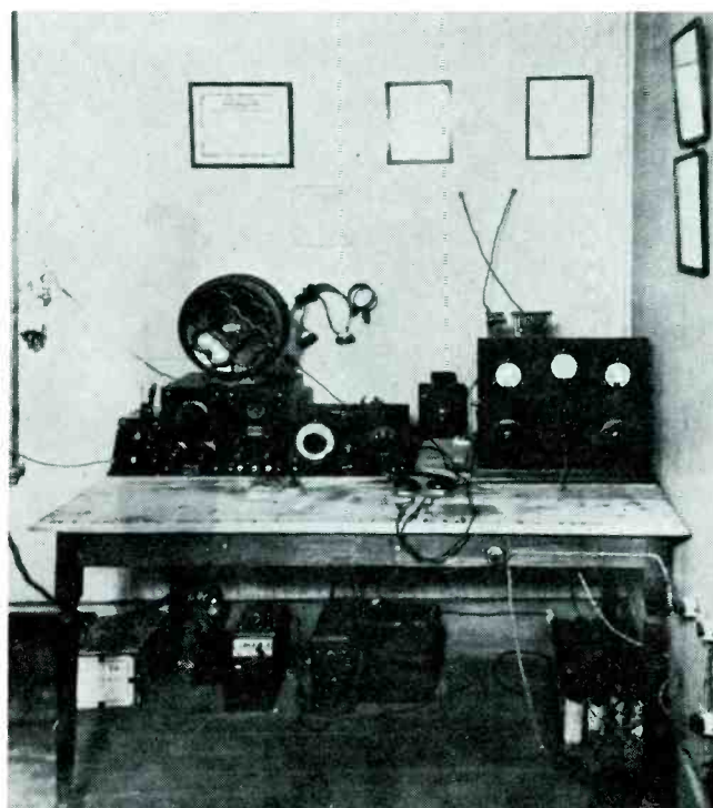
Fig. 3. A composite transmitter in use in 1919. Note the chemical rectifier on the floor at the right end of the table.
