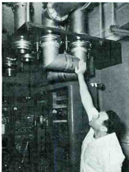
A "feel test" may be used to locate trouble in transmitter RF plumbing.
